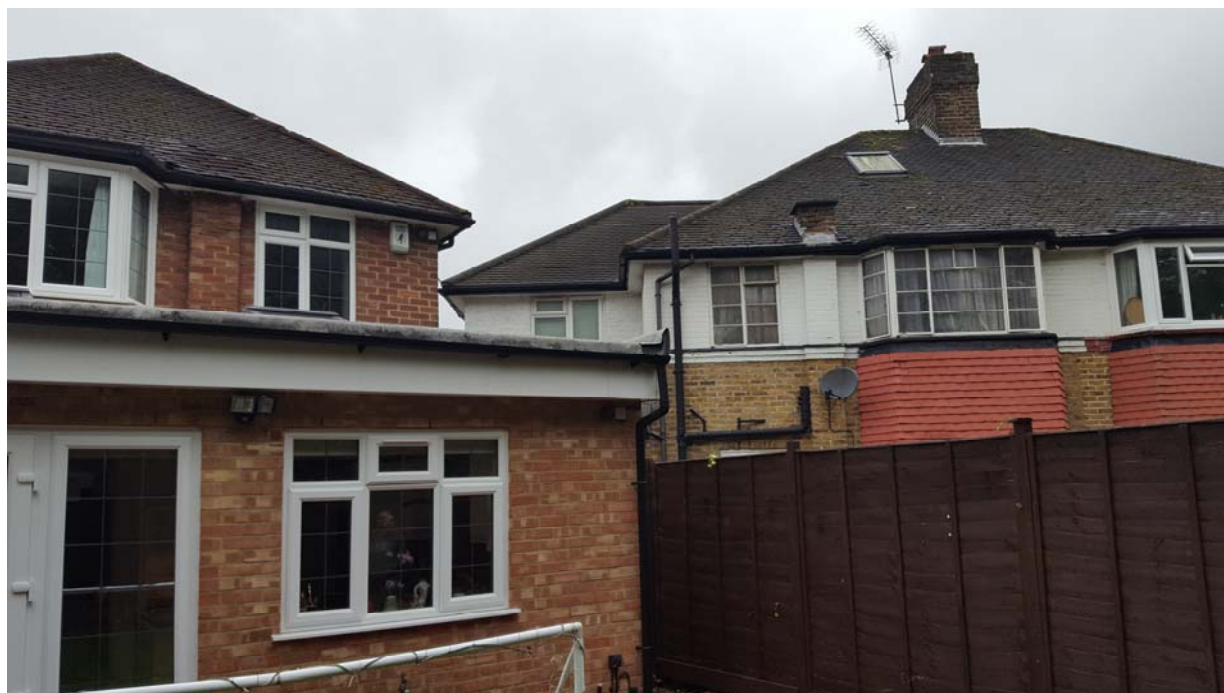
Rear elevation and view of neighbour at no. 102 Cheyneys Avenue
