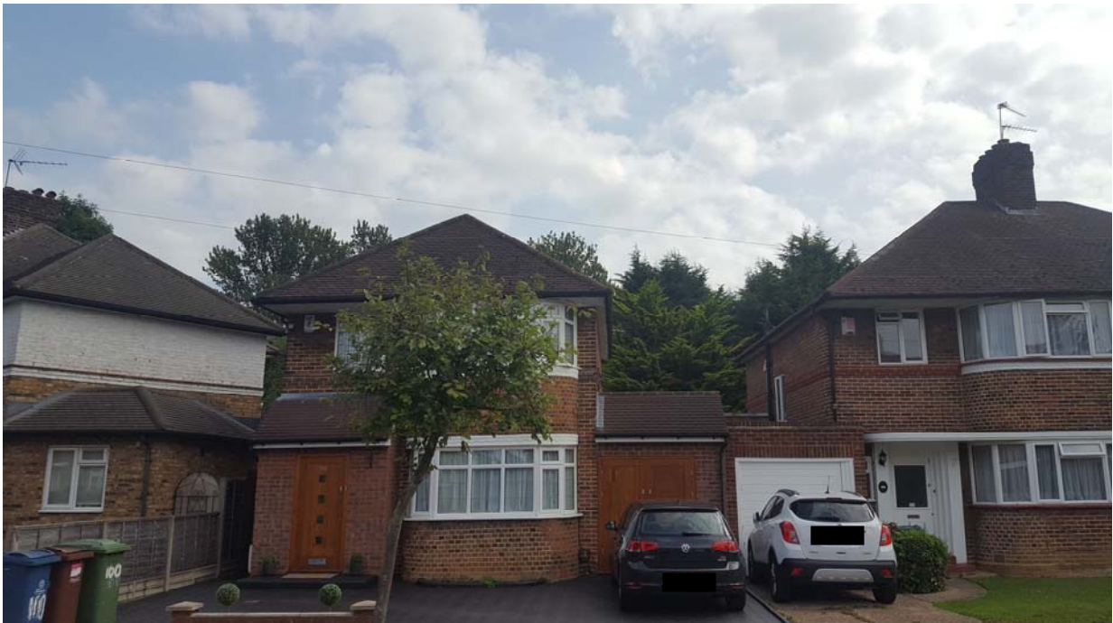
Gap between No. 100 and No. 98
