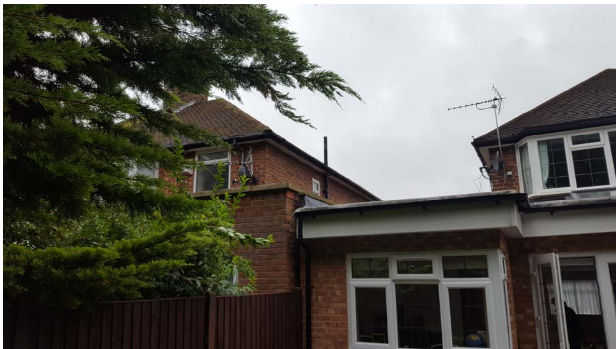
Rear elevation and view of neighbour at no. 98 Cheyneys Avenue
